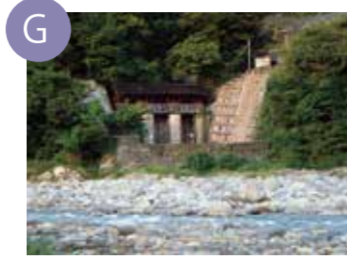
Water Channel Gate
